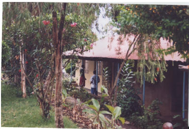
The roofs are now painted!
